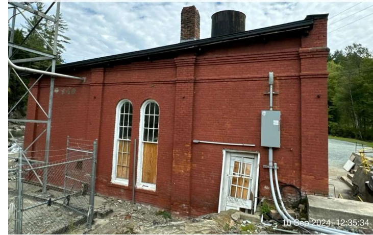
Photo 4: East elevation of the Wolcott hydropower building
