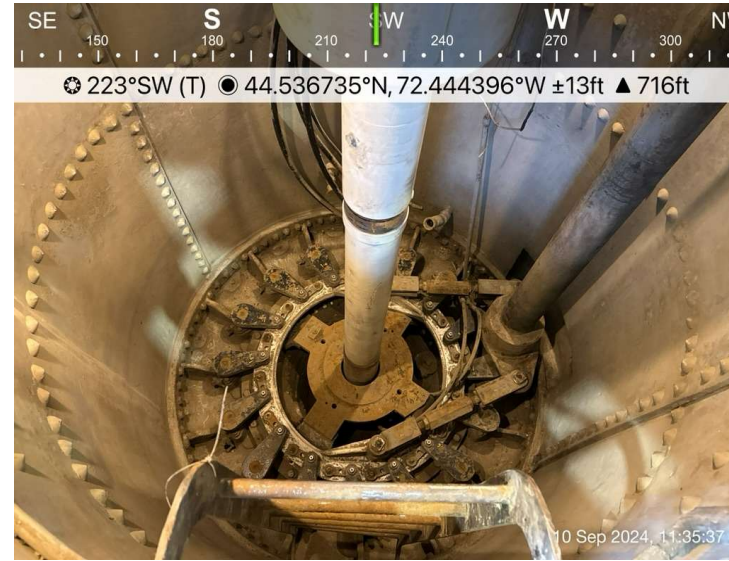
Photo 10: Detail view down into well / turbine area in September after July 2024 flooding
