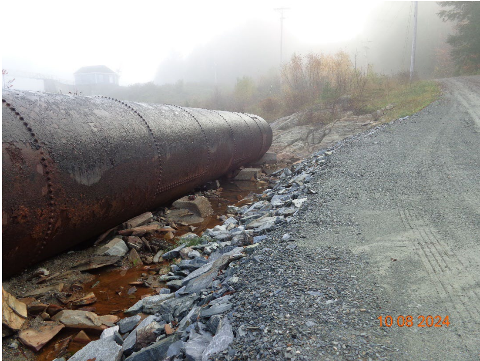
Photo 8 Looking up penstock at bend
